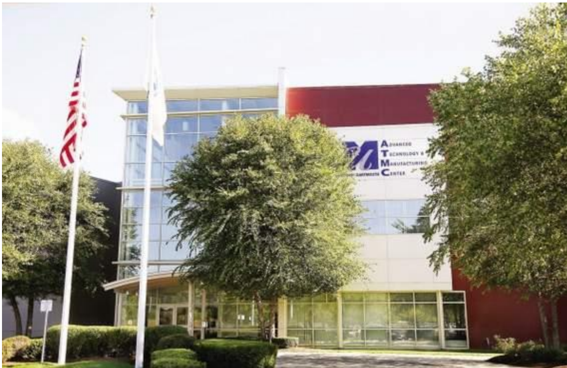
The Advanced Technology & Manufacturing Center, located at 151 Martine Street in Fall River
